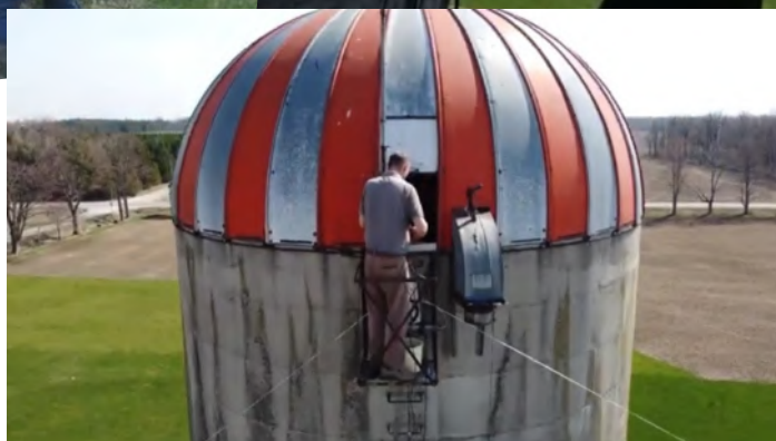
Preparing all the supplies and attaching the centre of the dipole at the top of the silo.
