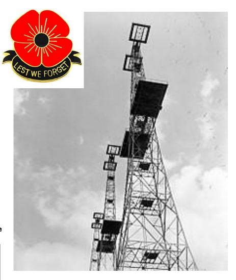
Three of the four transmitter towers of the Bawdsey CH (Chain Home, or CH for short, was the codename for the ring of coastal <u>Early Warning radar</u> stations) station as seen in 1945. The antennas proper are just visible at the extreme right. (Wikipedia)
