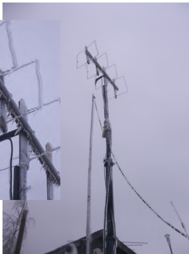
Yet the 2M quad beam withstood the brute force of the storm.
