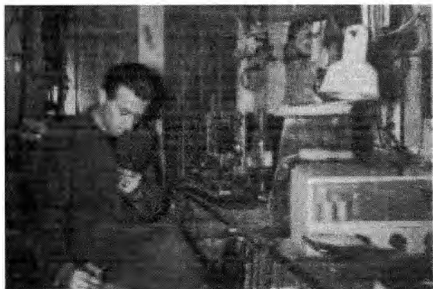
Fig. 3. Radio technician Hossfeld operating the telephone transmitter, which was quickly constructed using parts that were available, including the coil wrapped around the bottle in the center of the photograph.
