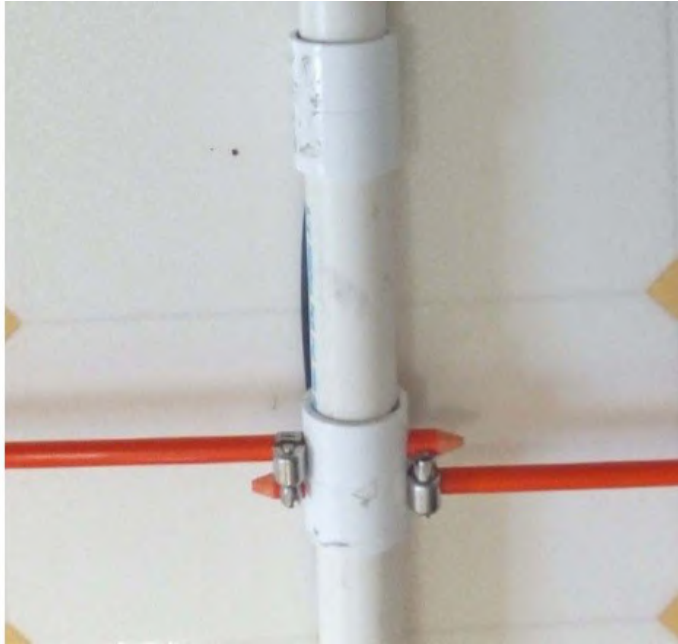
Fiberglass support rods pass through holes drilled in the PVC coupler. Hose clamps work as adjustable stops.
