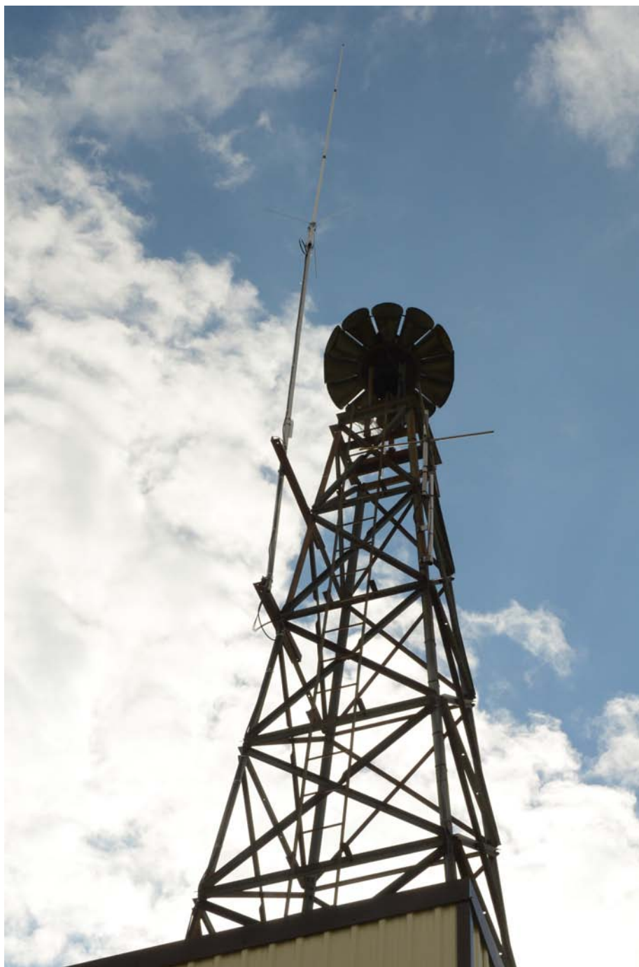
ERC antenna site at the Elmira Fire Station.
